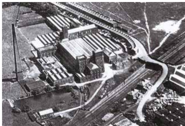
Farington Mill, with Mill Lane, home to many of the workforce, at the top of the picture. Note also the chimney which, at 225 feet tall, was a visible landmark for miles around
