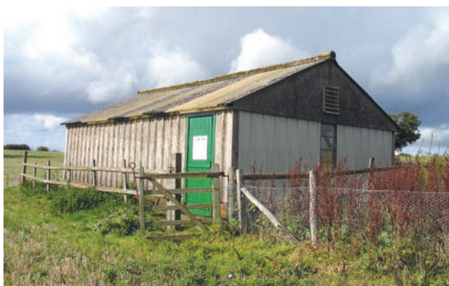
The hut built to protect the excavated pit-dwelling
