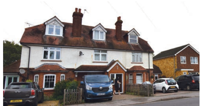
Beaver and Norton Cottages today. Beaver to the left of the two newer houses built on what was Alfred's vegetable garden, and Norton to the right. No. 1 Beaver Cottages (now known as 36 Send Road) has the white Toyota in front. 2 Norton Cottages (now known as 43 Send Road) is the centre property in the terrace
