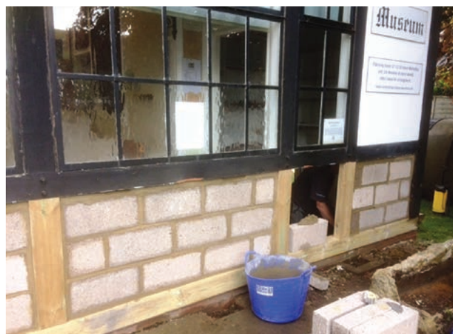
Rebuilding the front wall
