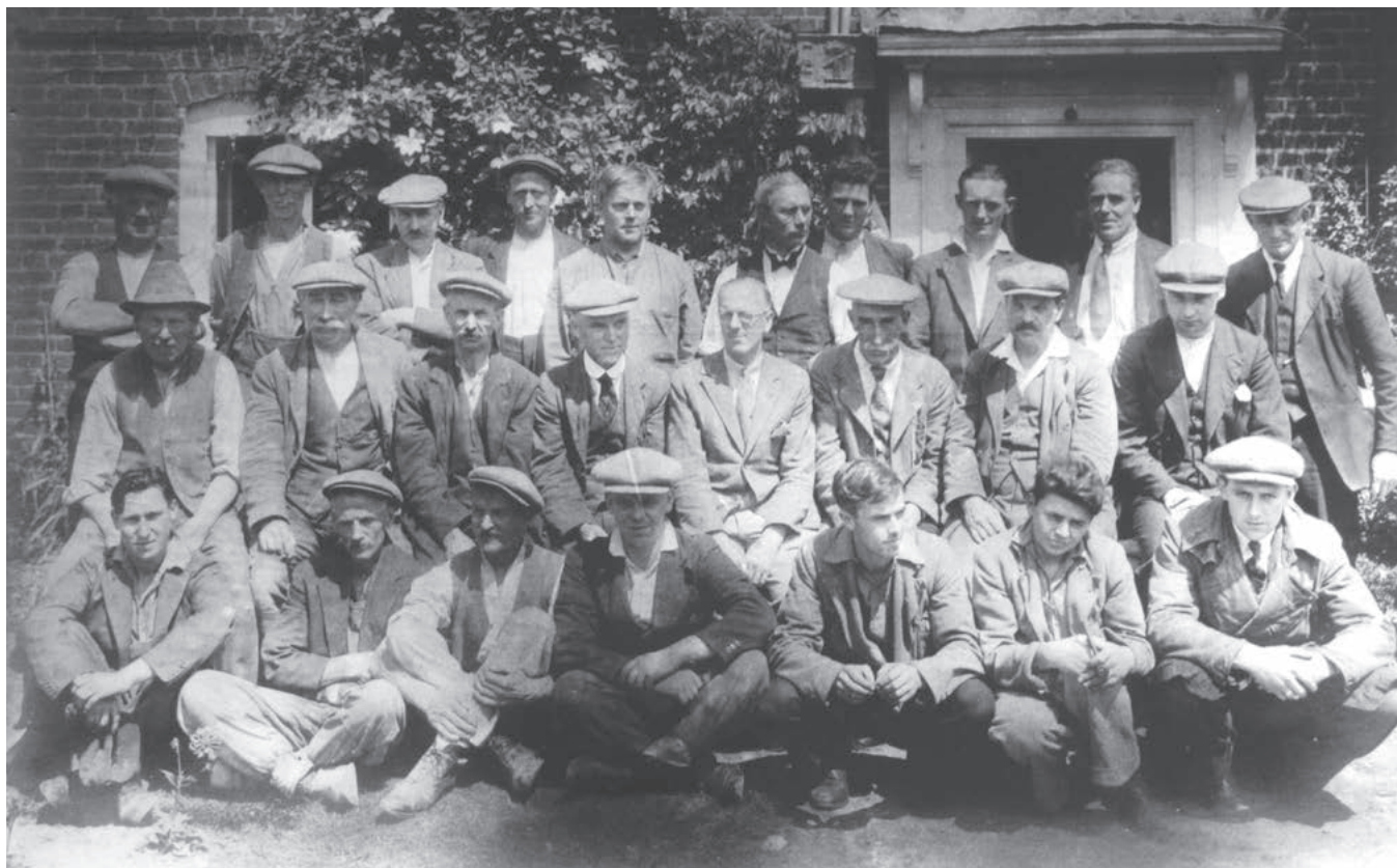
Bridge End in 1933 and the workforce who took part in the renovation works © Charles Hewlett collection
