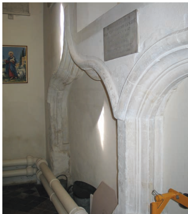
The early windows hidden behind the organ
