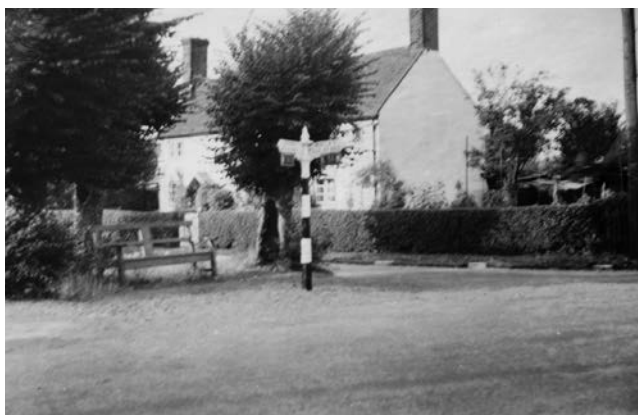
The corner of Send Marsh Green, with a pollarded elm tree in front of Bert's family home. When the tree was cut, nothing was wasted; the trimmings were used in the garden as pea sticks.
