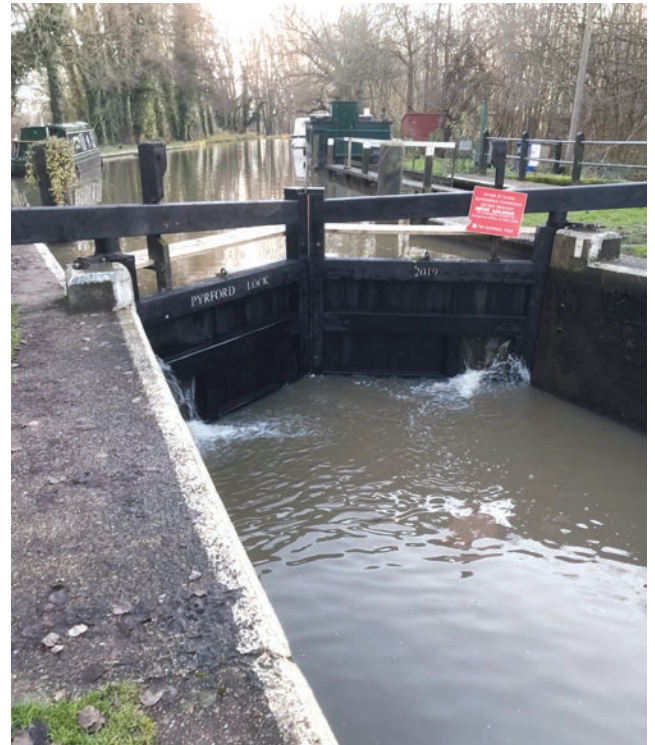
The new upstream gates
