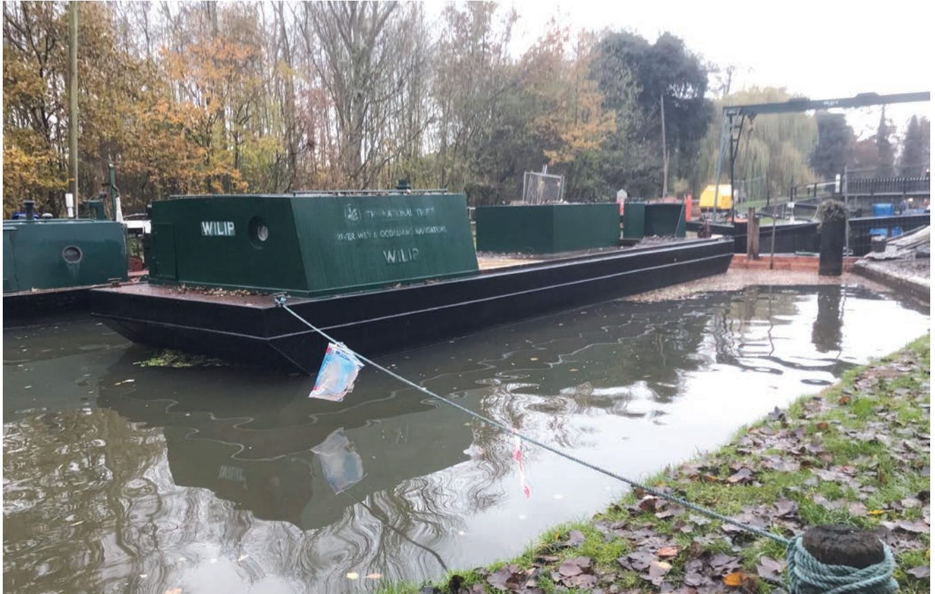
One of the National Trust barges used to transport the building materials to the site
