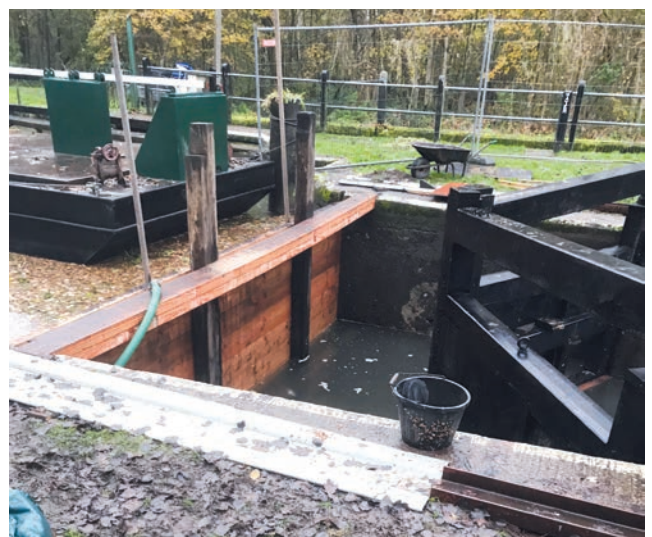
The dam is installed upstream of the gates
