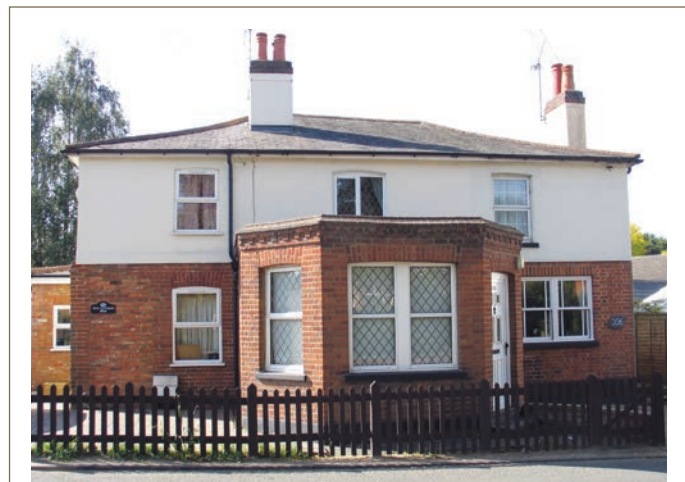
The site of the original Institute at 204-206 Send Road
