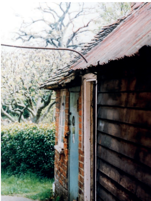
The two doorways taken from the front of the property (Send Road) in the 1970s, the far door being the entrance to the butcher's
