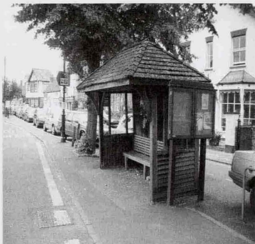
Ripley Bus Shelter Today
