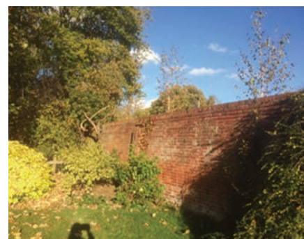
Part of the boundary wall that still remains and lies behind numbers 8 and 10 Heath Drive
