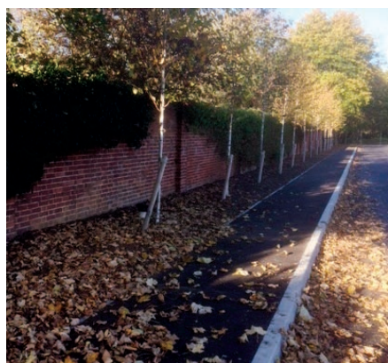
Part of the old boundary wall on Galileo Drive
