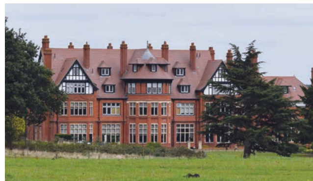
Hatchford Park – the roof has been much altered in recent years
