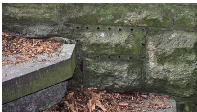
Top: The remains of the interior of the crypt – note the ventilation positions on either side of the window. Four more are located to the left and right behind the walls containing the coffins
