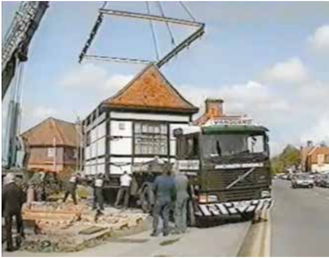
The old Nat West Bank building being lifted onto the back of a lorry
