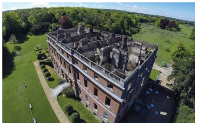
Aerial views showing the extent of the structural damage (photos NT)
