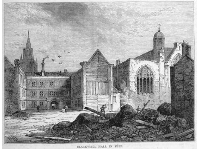
The Blackwell Hall being demolished in 1812 (courtesy Mechanical Creator Collection, Wikipedia)
