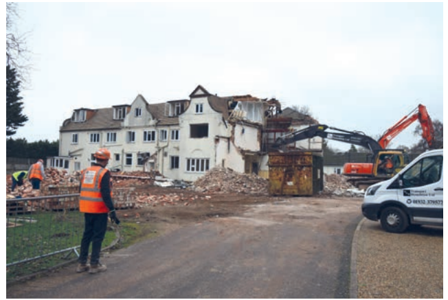
Demolition of Boughton Hall, November 2020 © Alan Cooper
