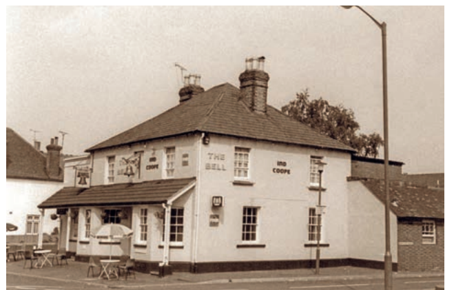
Top: The Bell, Stoughton, photographed very shortly before William Stansfield became landlord
