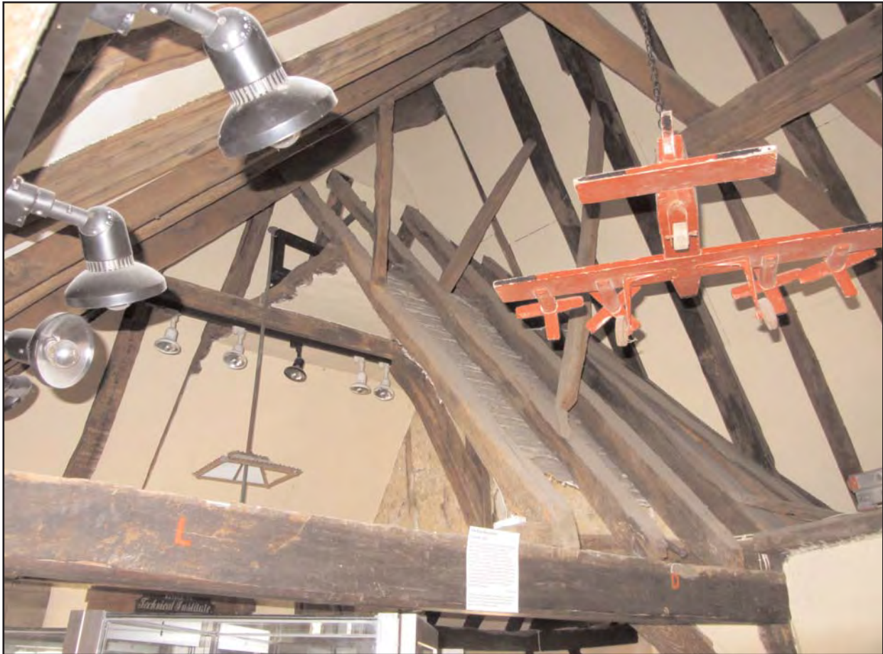
Inside Godalming museum showing part of the roof of the 1400s building with part of the woodwork attaching the Wealden house to it
